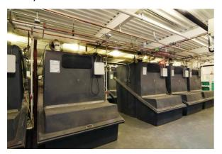
huge cost of tunneling under the Bronx River Parkway. Instead, the Zoo decided to install a Clivus Multrum Composting Toilet System consisting of 10 composters. In addition to saving money, the Clivus systems capture and recycle the nutrients in human waste and use only minimal water for flushing.
