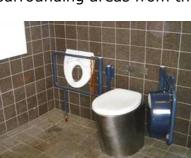
The toilets were built with stainless steel stools connected to Clivus Multrum units placed in the basement.
